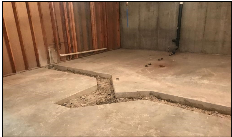
Piping covered in gravel and ready to fill in with new concrete.
