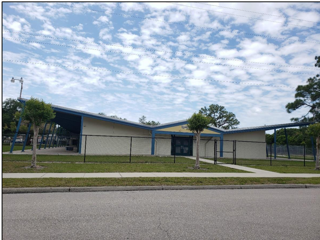
Figure 47: S002502, addition to the Alta Vista School, located at 1000 South School Avenue.
