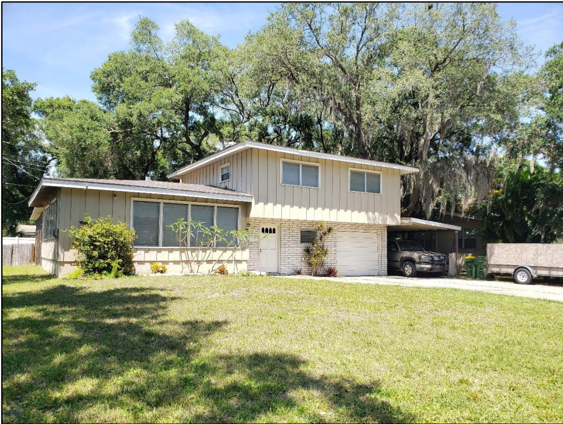
Figure 41: S011433, 3117 Alta Vista Street.
