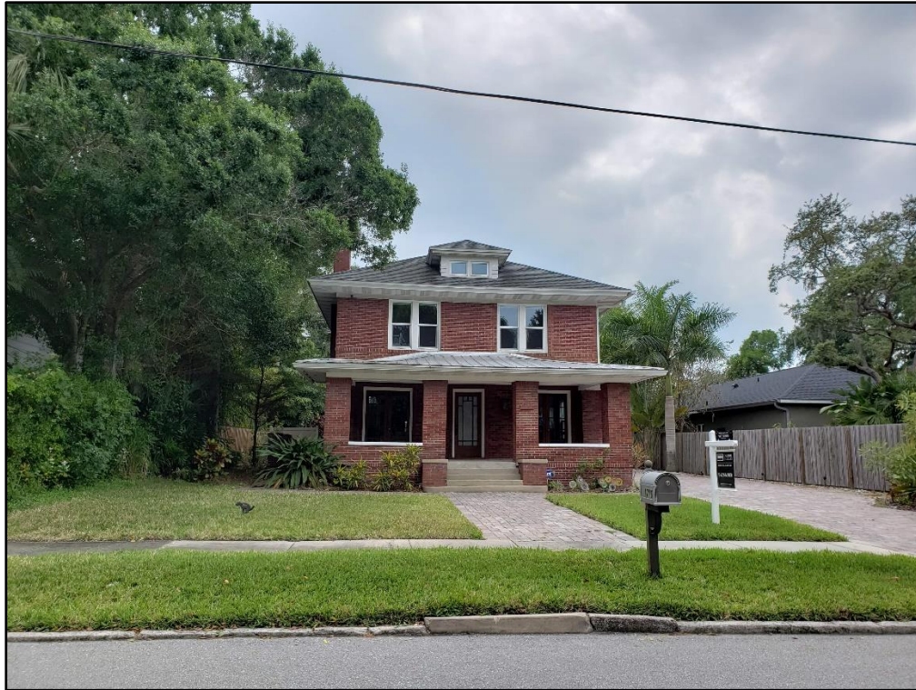
Figure 51: S000737, 1716 Hawthorne Street, shows the Prairie style of Architecture.
