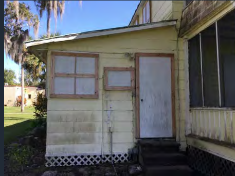
1700 Vamo Drive rear (North) – showing one story wood wing on the west side of rear façade. Not know if this is an addition or original to the property, but it shows in the next old photo.
