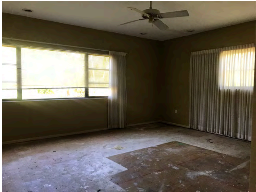
Note Wood Floor under Tile
