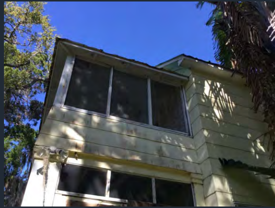
1700 Vamo Drive – West side elevation continued, showing 2 nd and 1 st floor Sun Porch.
