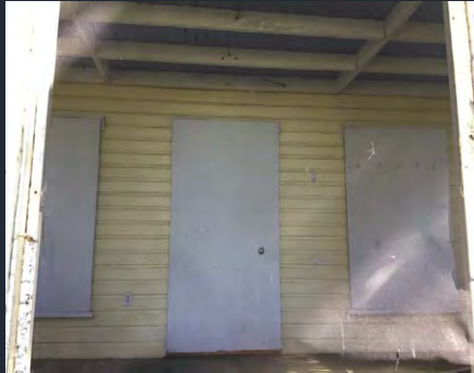
1700 Vamo Drive Rear (North) Elevation inside the sunporch. Novelty siding and center door entrance. This wood siding was apparently covered by Asbestos siding popular between 1906 and was banned in 1978.
